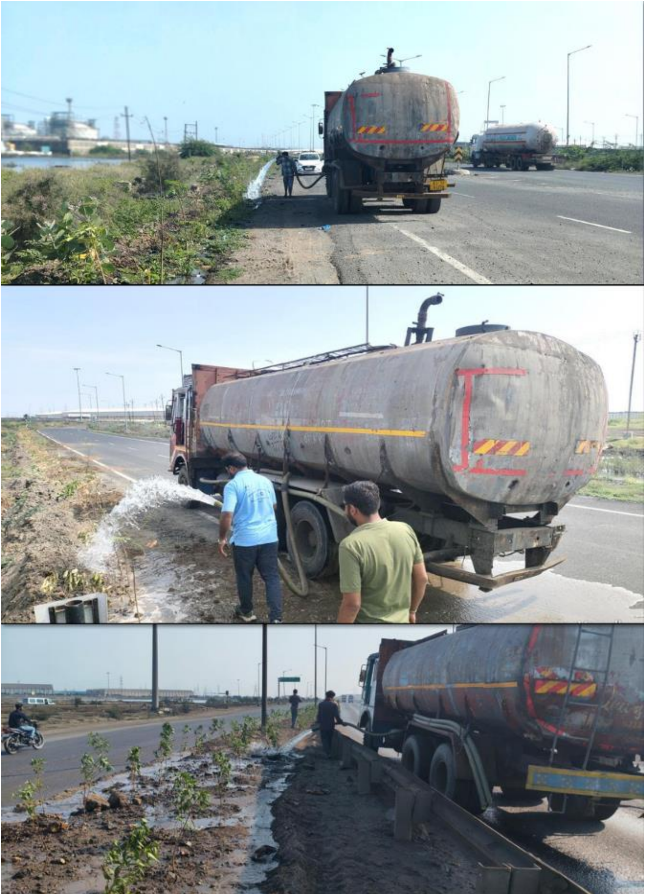
Plate 6: Watering in progress
