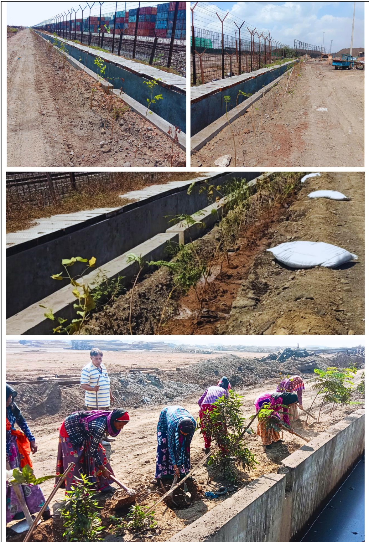
Plate 1. Soil and moisture conservation works carried out at the plantation site
