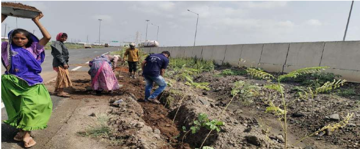
Fig. Fertile Soil Filling to the pits
