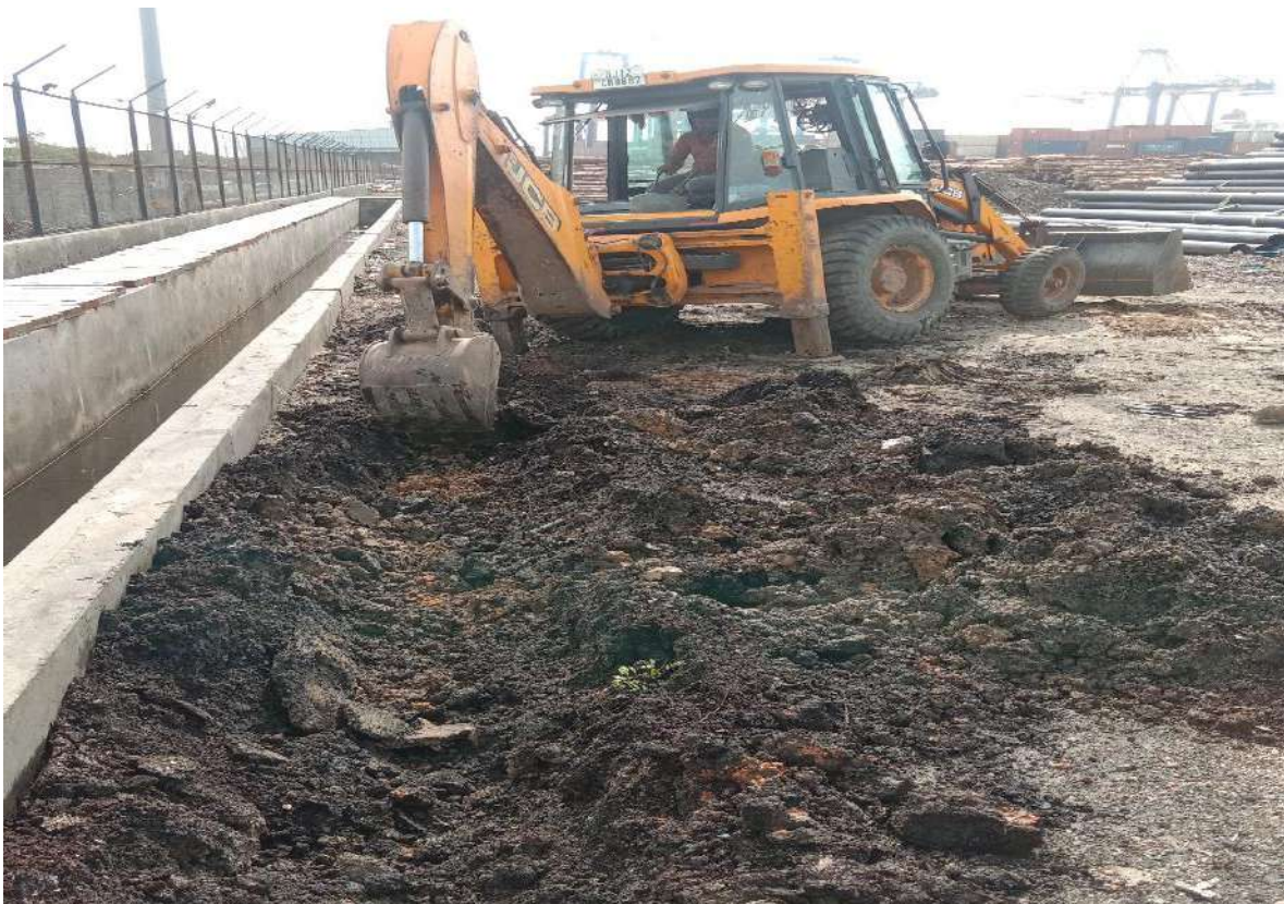
Fig. 3 Digging Out Trench for Plantation
