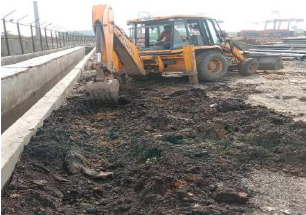
Fig. 3 Digging Out Trench for Plantation
