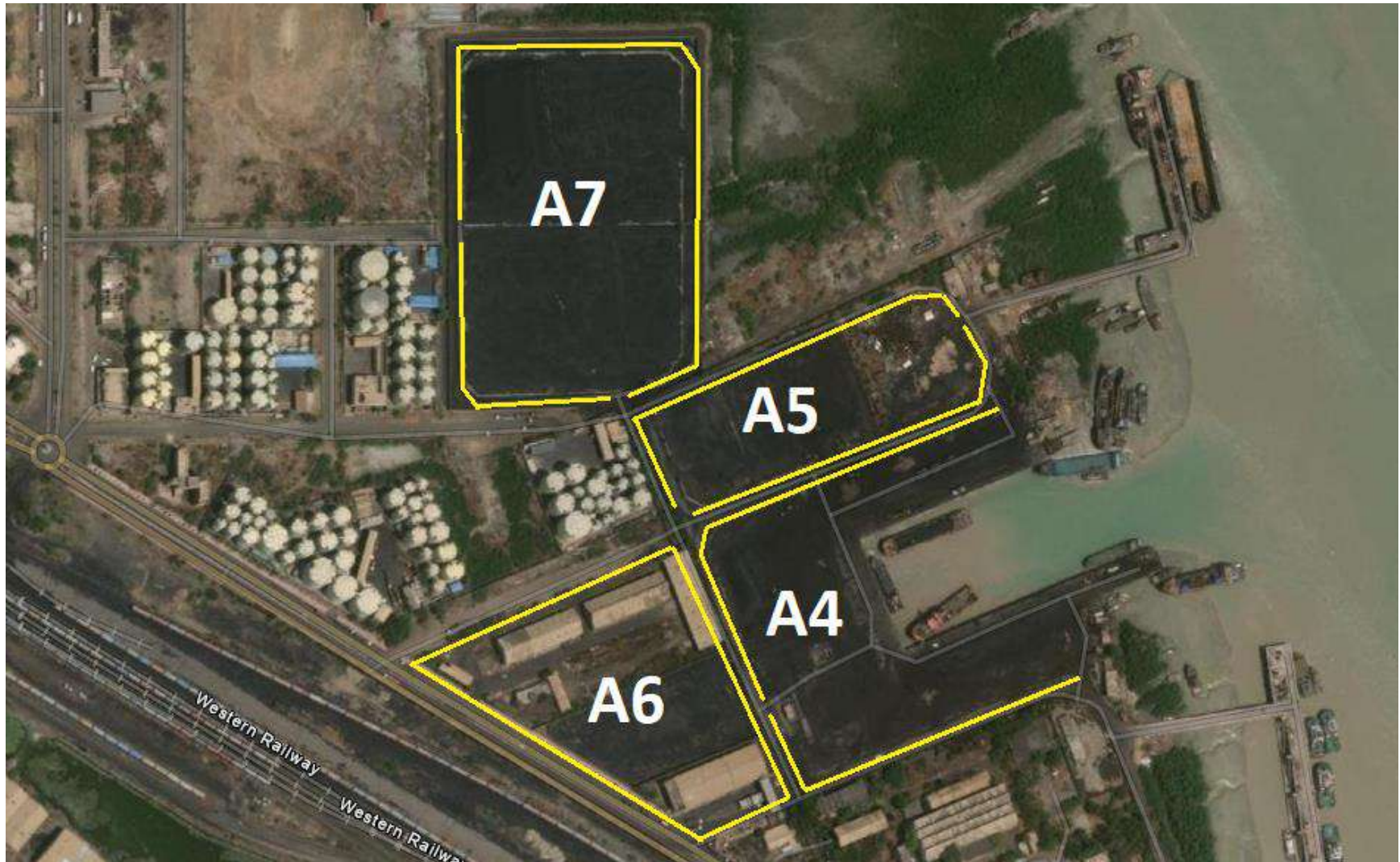
Fig. 2.5: Demarcation of plots in Coal Handling and Storage Area
