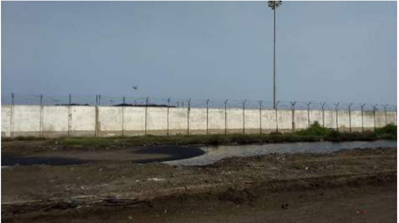
Fig. 7.5: Compound wall along coal yard periphery
