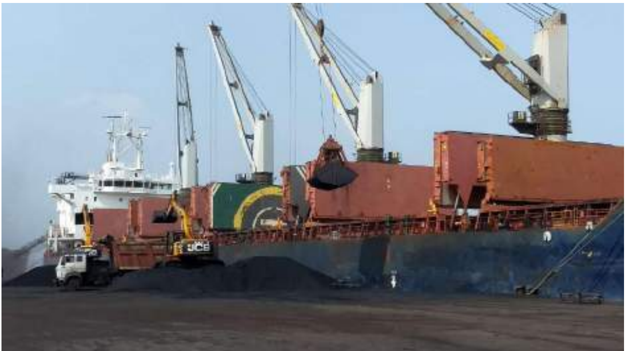
Fig. 7.1: Unloading of coal on wharf floor with the help of grab and subsequently to dumper through JCB machine
