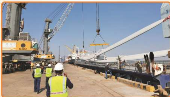
Handling of Wind Mill Blades of length 83.3 Meters at DPT.
